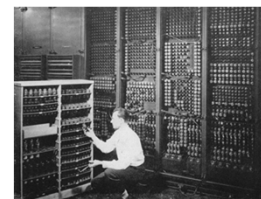
Replanning a ball tube socket (stacking) among ENIAC's 15000 switches.
